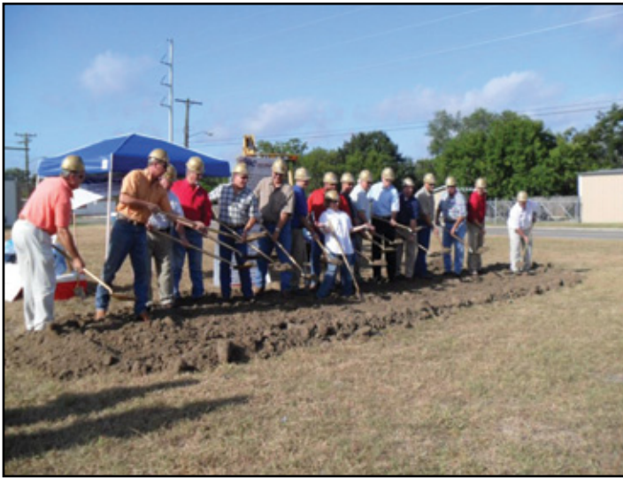
On August 16th, the Past Board Chairmen and current Board of Directors and members of the ABC Mid Coast Chapter came together with gold hard hats and gold shovels to break ground on the site where the Chapter's new building will be built.
